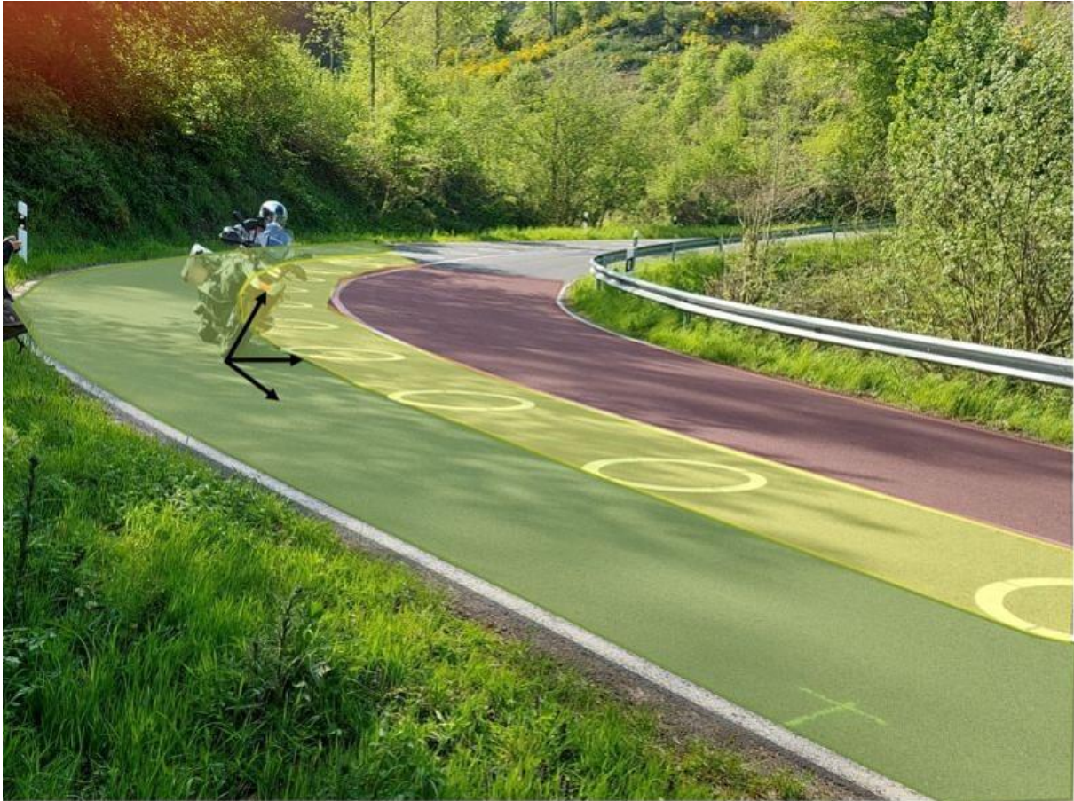
Figure 2. Division of the road in three different zones according to their safety level
