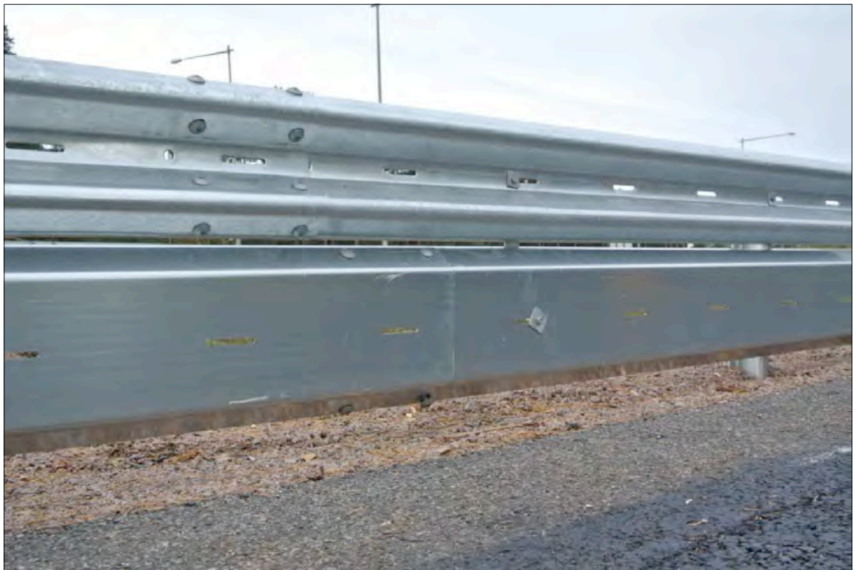
Picture 3. W-profile barrier with MPS, installed on an exit of E4 outside Gävle 2014.
