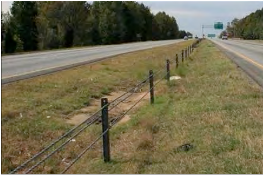
Picture 1. Median cable barrier installation in USA
