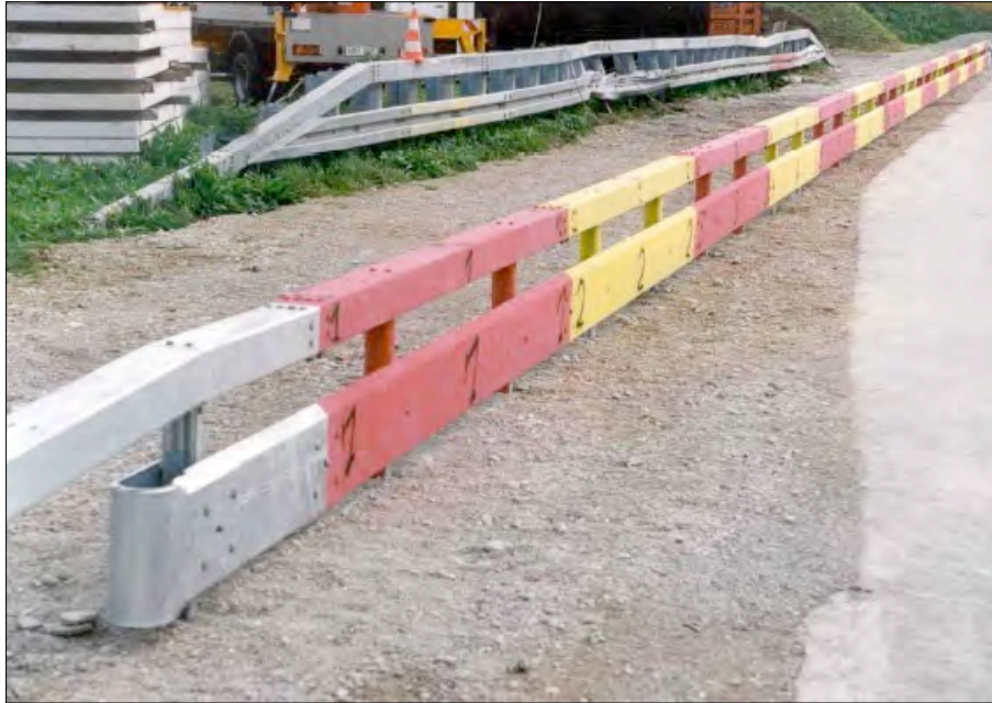
Picture 3. Box beam barrier with MPS, Germany.
