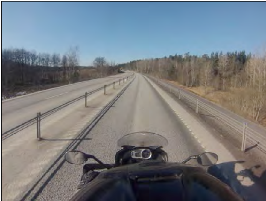
Picture 2. Cable barrier installation 2+1 in Sweden (Finspång-Norrköping).
