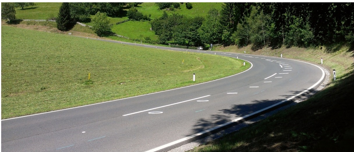
Figure 10. Elliptic floor marking
