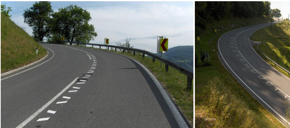
Figure 2. First application of floor markings, B69, „Soboth“-Route 1 . Source: Höher, 2012.
