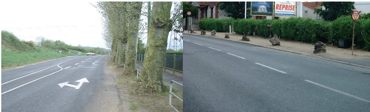
Figure 9: Obstacles (trees and rocks) on the shoulder of the road which can cause more serious injuries
