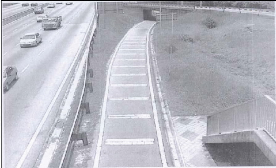
Separate ride-way along Federal Highway, Route 2. (Picture: Radin Umar, Law Teik Hua)
