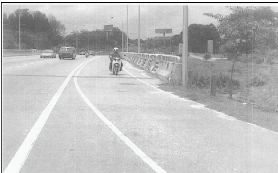
Inclusive/non-exclusive motorcycle lane along Federal Highway towards Subang International Airport. (Picture: Radin Umar, Law Teik Hua)
